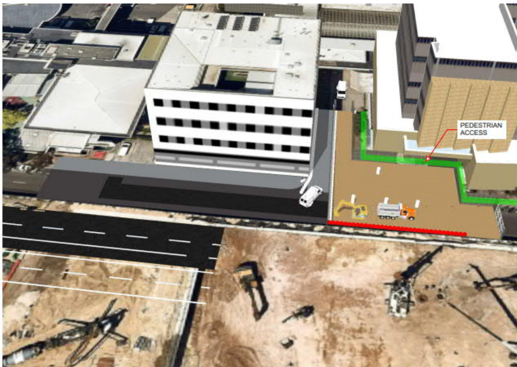
Figure 10 – South stage – Bulk excavation– stage 4 of 6
