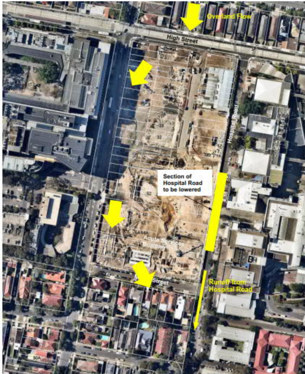
Figure 1 Location of Hospital Road works
