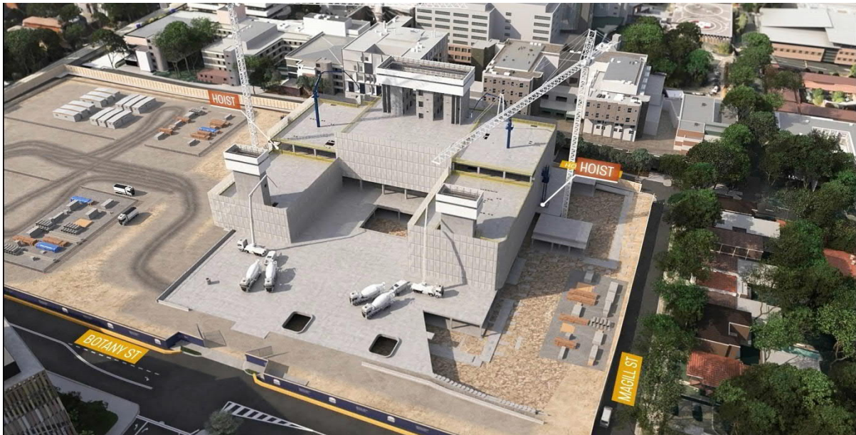
Figure 10: Crane and materials hoist
