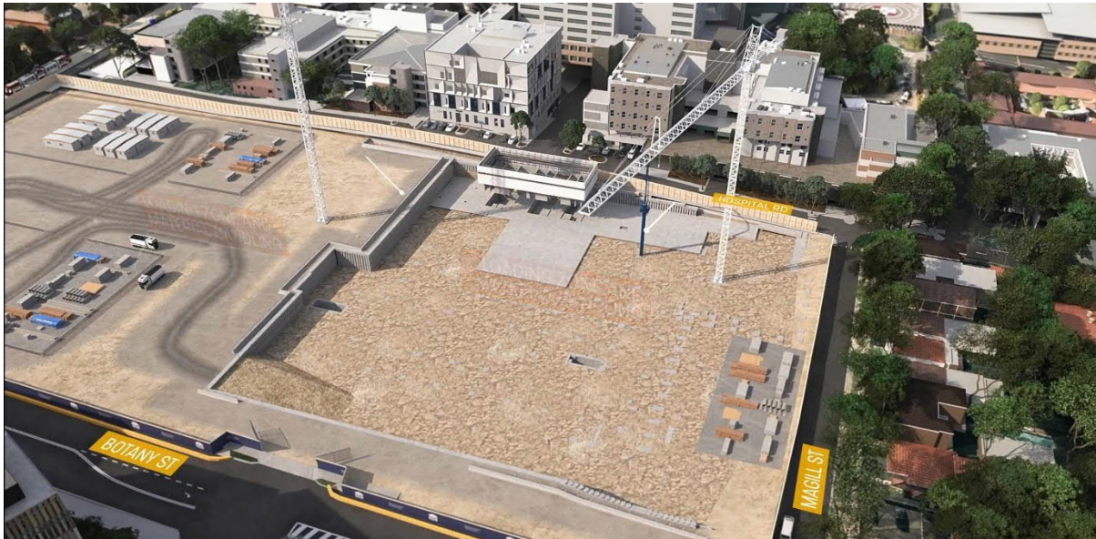
Figure 9: Crane and materials handling
