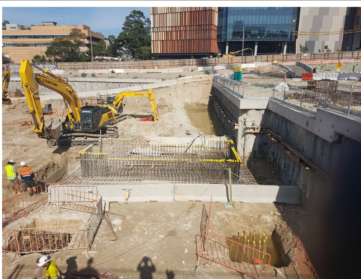
Current main work area – detailed excavations and preparation for one of the building cores
