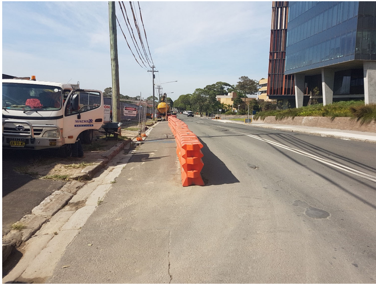
Partial lane closure on Botany Street in preparation for the relocation of the HV line (Ausgrid works)
