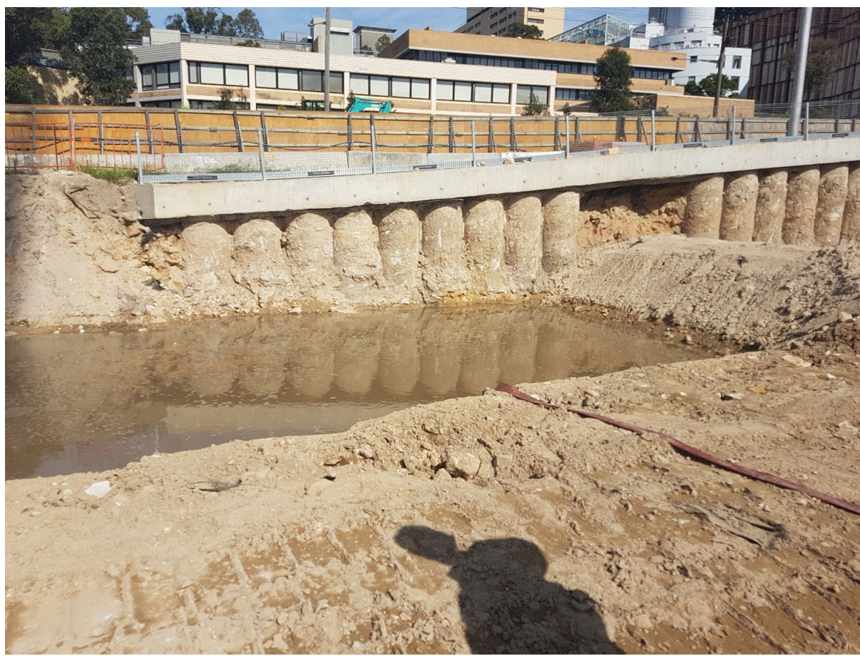
End of line stormwater detention basin
