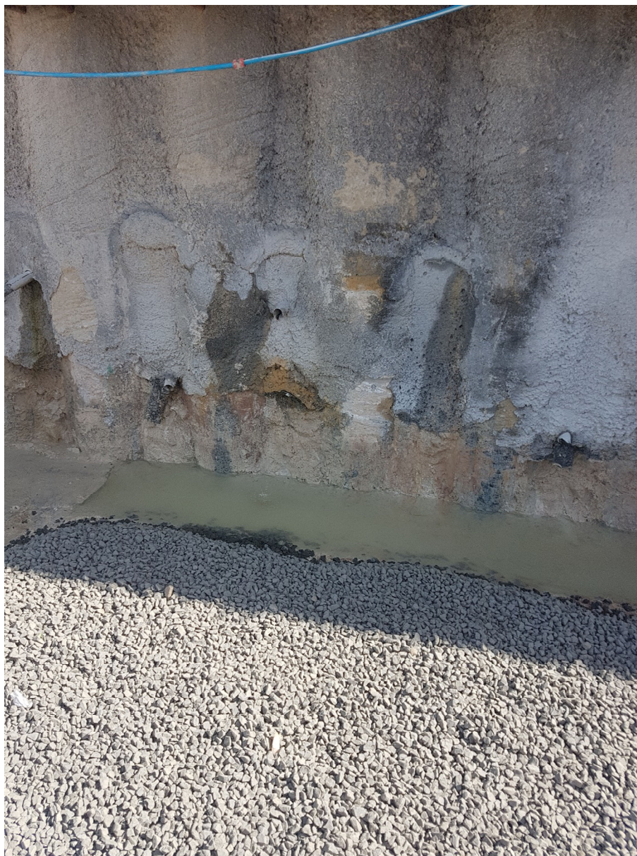
Area of groundwater infiltration. The groundwater in this area appears to flow constantly, as opposed to other interceptions which flow only after rainfall
