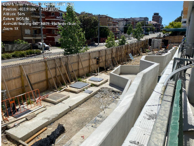
Photo 11 – Permanent floodwall, covered stormwater pits and areas for landscaping.
