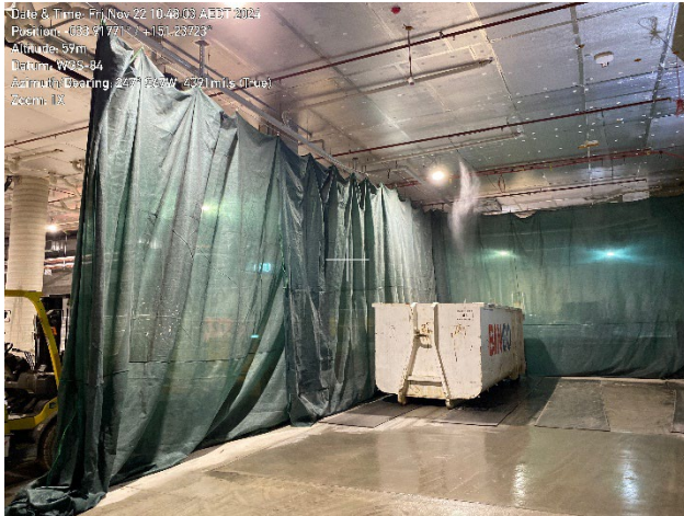
Photo 1 - Waste skip bin on floor B2 with sprinklers and dust curtains to reduce dust impacts adjacent to the bin during filling.
