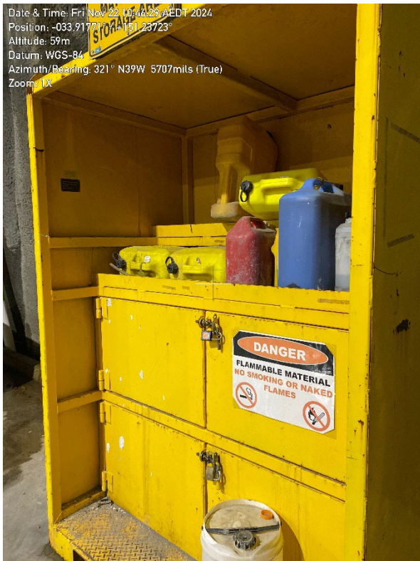
Photo 17 – Flammable liquid storage cabinet on level B2.
