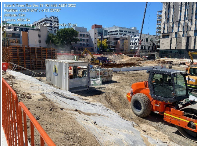
Compacted soil in the background. Geotextile-lined soil in the foreground. Waste station with receptacles in the centre of the image.
