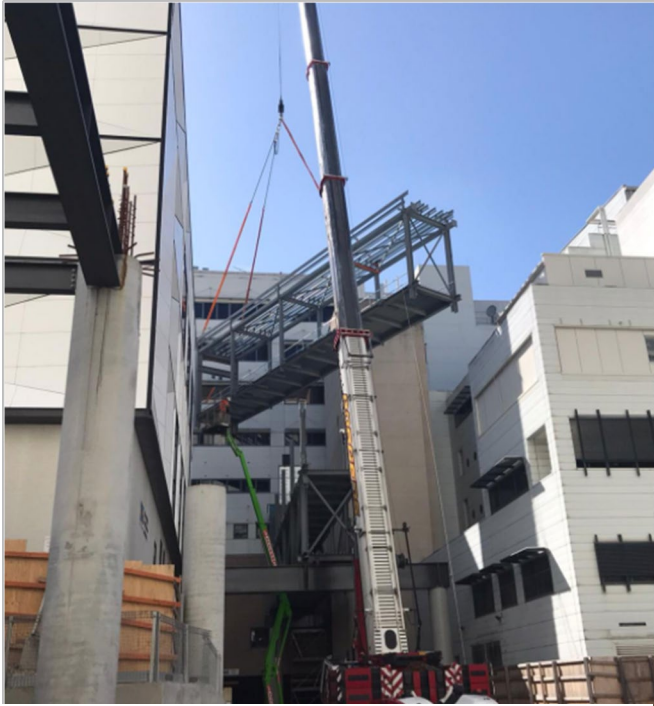
Installation of link bridge modules for the patient link bridge
