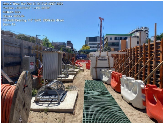
Covered pits and hoarding. The blue noise blanket erected on the hoarding can be seen in the background of the image.
