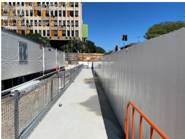
Fenced walkway within the site and the flood protection wall erected along High Street (pictured right).
