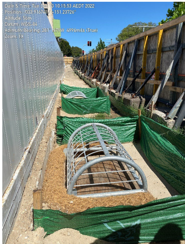
Covered pits along High Street with sediment controls. Located between the site hoarding and the flood protection wall.
