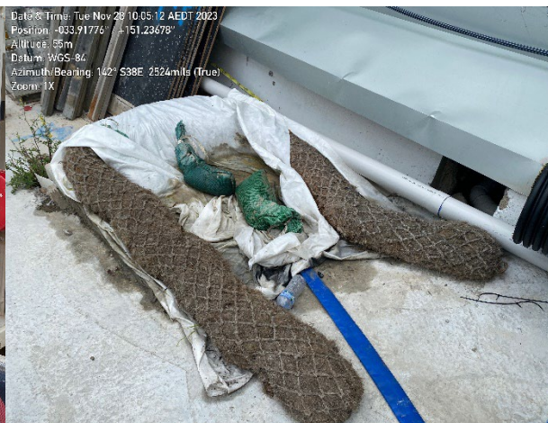
Nurse station adjacent to temporary driveway. Covered drain surrounded by a coir log Coir logs lining temporary driveway to mitigate dirty water runoff beneath the concrete divider. adjacent to site temporary driveway from Botany Road.
